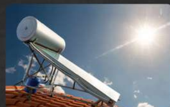
Solar Water Heater
